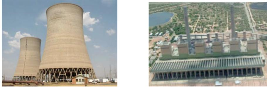
**Figure 6-4. Eskom's dry cooling towers at Grootvlei (Indirect system with surface condenser and dry cooling tower) and Matimba air cooled condenser dry cooling. (source: Eskom)**
