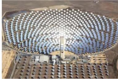
**Figure 4-19: Solar Thermal Power Plant. Power Tower Type**
