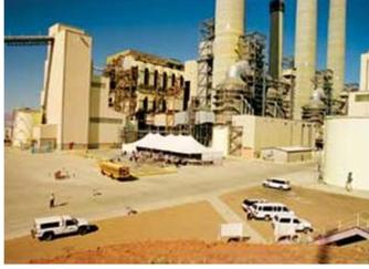
**Figure 7-2. Navajo Generating Station (NGS), situated in northern Arizona near the Grand Canyon, a water-scarce area. It uses a zero-discharge water treatment process: all cooling tower blowdown, all wastewater, and most storm water are recovered, recycled, and reused in plant processes (Source: NGS website)**
