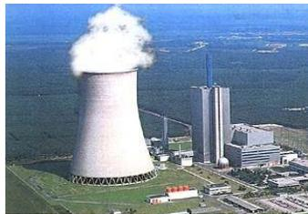
**Figure 2-8. Picture of a natural draft cooling tower**
