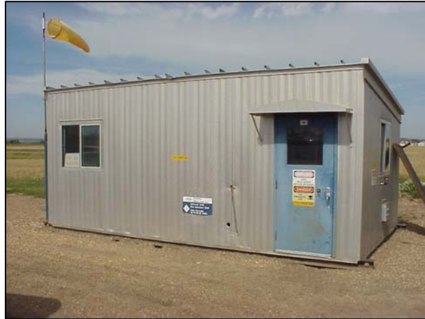
Figure 3.2: Acid Gas Injection Well House, Acheson Field (Photo taken by the author August 29, 2002, courtesy of EnerPro Midstream Inc.)
