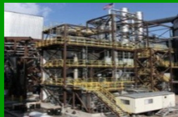
WE - Energie USA WI - 5 MWth Chilled Ammonia, Coal
