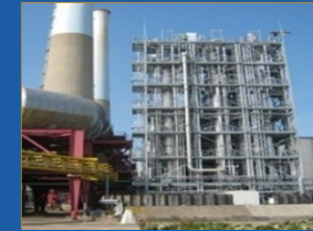
EDF Le Havre France - 5 MWth Adv. Adv. Amines - Coal
