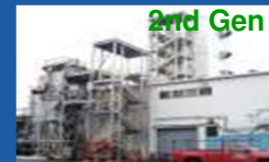
DOE/Alstom Windsor US - 3 MWth Chemical Looping, Coal
